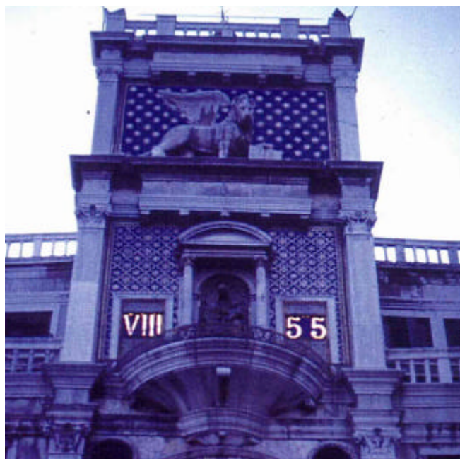
6. The panelled wheels viewed at night. The openings in which they are displayed are also used for the procession of the Magi, when the digital display is lifted out of the way.
